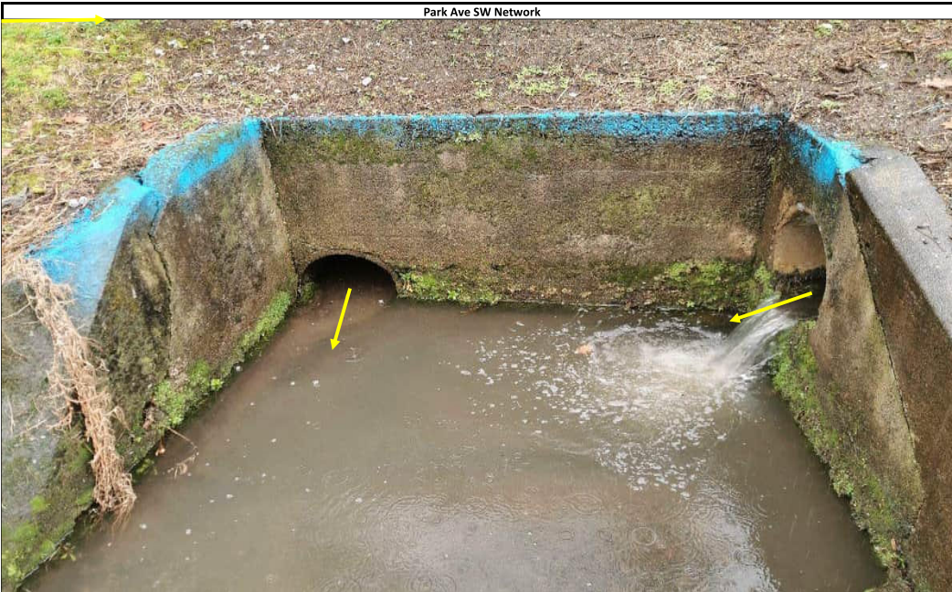
Photo 37 - Concrete Inlets around wingwall
