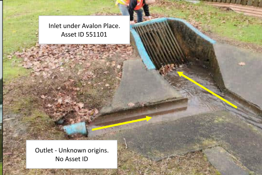
Photo 30 - Concrete Lined SW Channel View to North West
