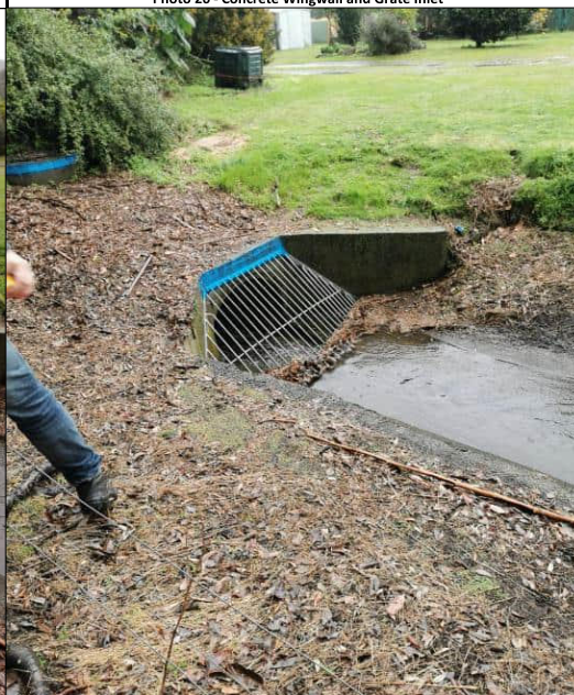
Photo 28 - Concrete Wingwall and Grate Inlet - DN900mm Concrete Inlet
