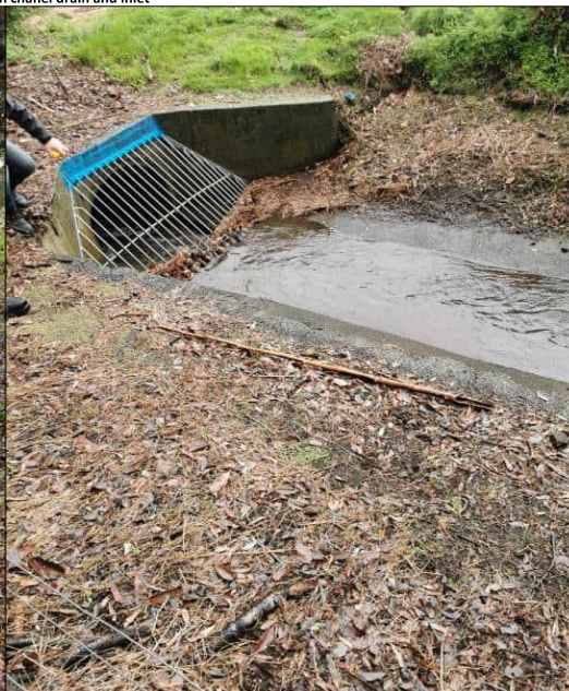
Photo 26 - Concrete Wingwall and Grate Inlet
