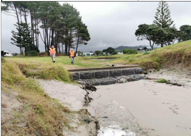
Photo 6 - Weir outlet for SW Pond view to Pond - Gabian baskets are 4x levels
