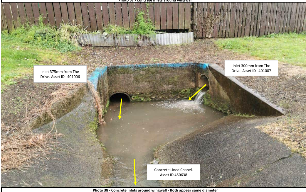
Photo 38 - Concrete Inlets around wingwall - Both appear same diameter
