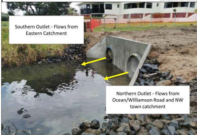
Photo 0 - New 2019 Project - Twin outfall to pond
