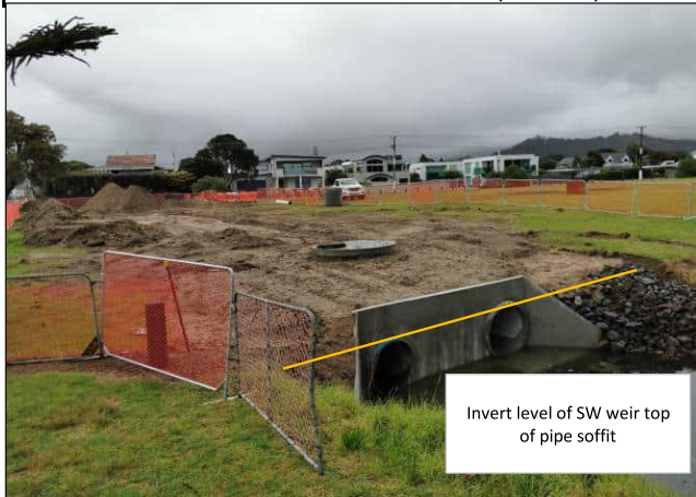
Photo 10 - New 2019 Project - Twin outfall to pond and manhole chamber
