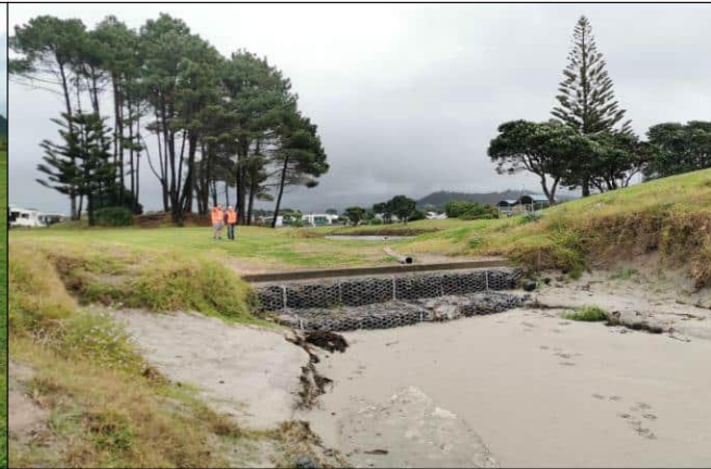
Photo 5 - Weir outlet for SW Pond (South West) - Gabian baskets are 4x levels
