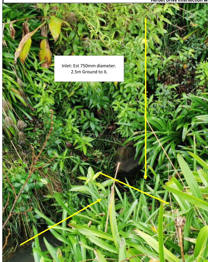
Photo 51 - Estimated 750mm diameter. 2.5m below ground level (invert)
