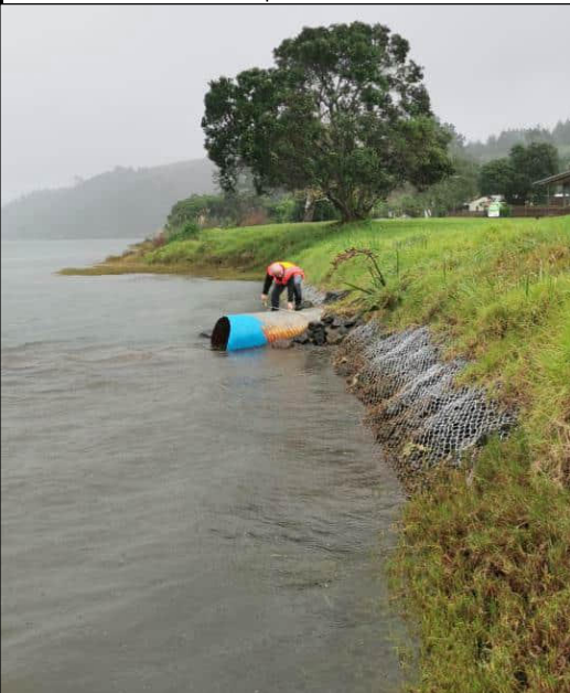
Photo 24 - Outfall photo for Asset ID 553249 - DN1000mm Corrugated Steel
