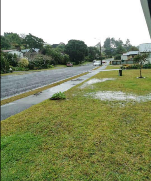
Photo 29 - Commonly flooded road section between catchpits 201289 & 300722
