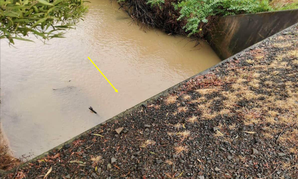
Photo 43 - IL 3.5m less than road. 2m culvert height. 1.5m cover
