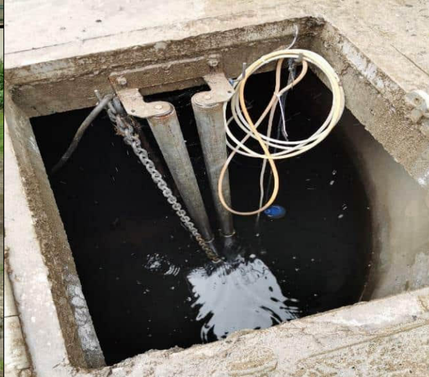
Photo 19 - Otahu SWPS Wetwell - Northern Chamber - 2 Pumps
