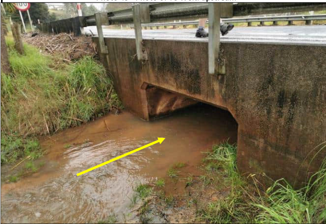
Photo 47 - 200mm blockage with sediment
