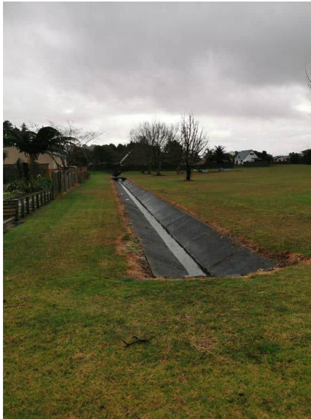
Figure 2-6 Concrete lined open drain at Park Avenue Reserve
