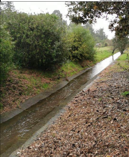
Photo 25 - Concrete Lined Stormwater Drain
