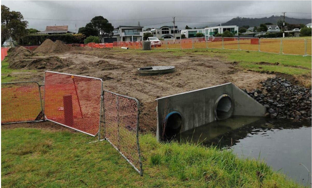
Figure 2-7 Recent duplication of SW outlet into Williamson Park pond
