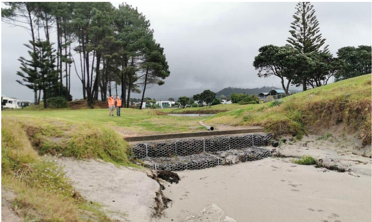
Figure 2-8 Gabion basket and concrete nib overflow from Williamson Park pond onto beach
