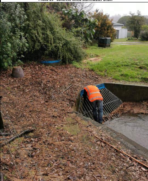
Photo 27 - Concrete Wingwall and Grate Inlet-Manhole above
