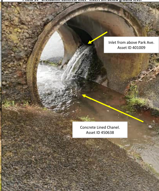
Photo 36 - Inlet 300mm Concrete from Western direction
