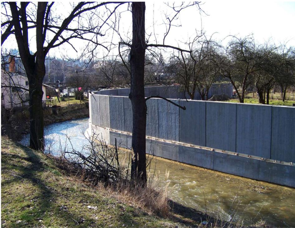
*Figure 10: Example of vertical concrete walls lining a stream*
