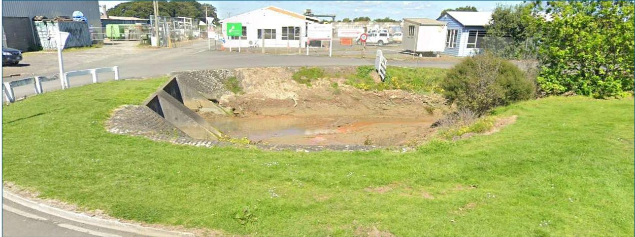
*Figure 37: Head of exposed drain - limited space and erosion prone with the culverts and drains requiring one-way flow valves*
