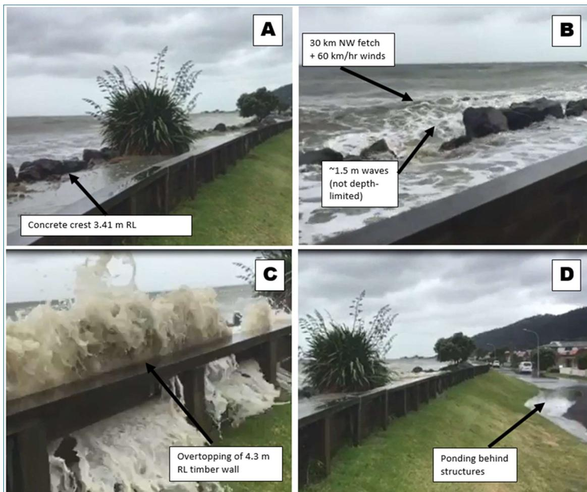
**Figure 6:** Waves overtopping Moanataiari defences on the 5 January 2018 (Note levels indicated are m MVD53)
