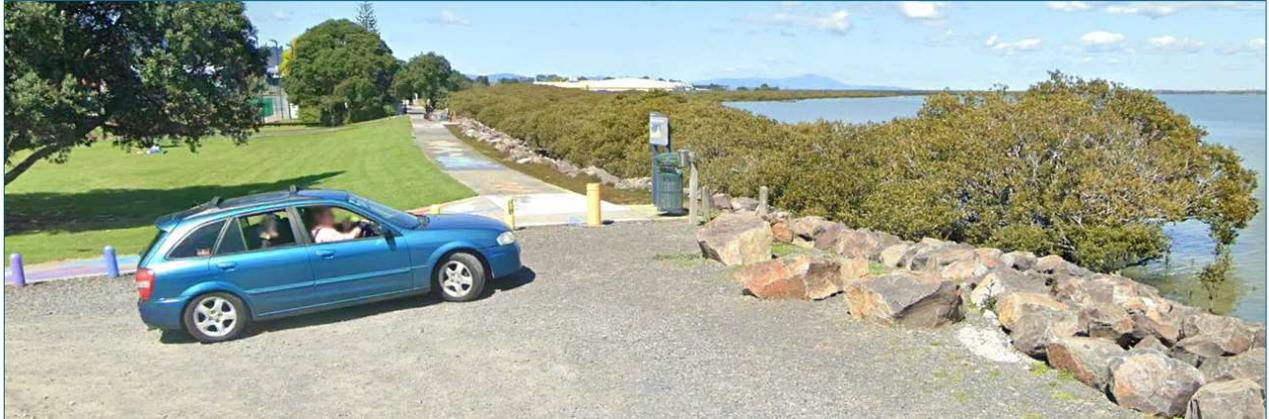
**Figure 35:** Low armoured bund protecting northern foreshore (at the end of Albert Street)
