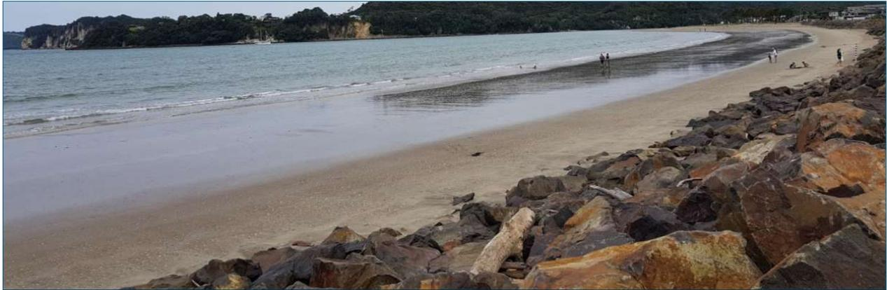
*Figure 15: Ocean facing armoured foreshore (Mercury Bay)*
