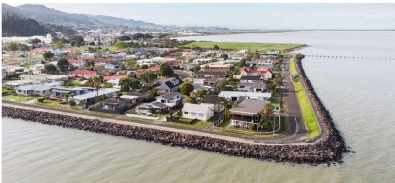
*Figure 7: Example of an armoured embankment face. Example from Moanataiari*
