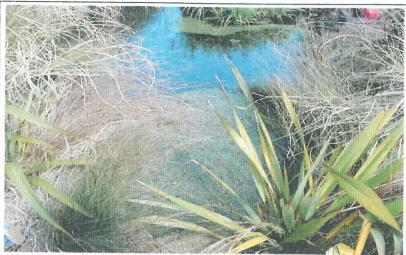
99340 Casement Road Open Drain Open drain within industrial area that flows toward the estuary mangroves. Culverts under crossings 50% blocked with sediment and rubbish. No bank erosion as banks are heavily vegetated.
