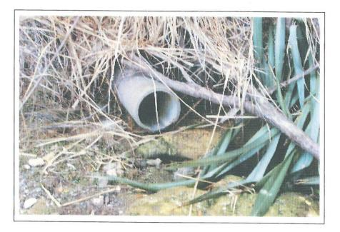
26720 Off Tukere Drive 300mm concrete culvert Concrete culvert outlet in good condition. SW flows directly into harbour. No erosion or sedimentation evident.
