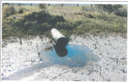
102871 End of Beach Road near proposed marina 300mm corrugated iron culvert Outlet exists at road level. Bank is vegetated and no erosion exists. No sedimentation exists within the culvert. No rock support is around the outlet for support.
