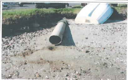
102866 End of Harbour View Road 300mm concrete culvert Outlet is at beach level with a 0.5m bank behind to the road level. Bank is vegetated with no sign of erosion. The end of the culvert is chipped at the outlet. No rock support exists around the outlet but is not required. No sedimentation evident.
