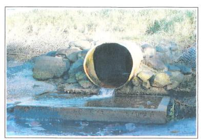
50820 Kotuku Street 1000mm corrugated iron culvert SW flows into concrete spill basin before reaching the beach. Concrete7d rock around outlet. Banks are stabilised by rock riprap in wire netting. SW has strong sulphur smell. No erosion around outlet or sedimentation in culvert evident.
