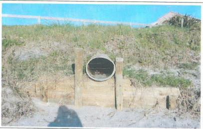
**ASSET NUMBER:** 50976 LOCATION: Off Pohutakawa Crescent **CULVERT SIZE:** 375mm concrete culvert CONDITION: Culvert outlet is supported on top of a low timber retaining wall which acts as a cradle. 3x horizontal steel grates are at the outlet. No sedimentation within the culvert or erosion around the outlet is evident. The surrounding banks are vegetated/stabilised with dune grass. None
