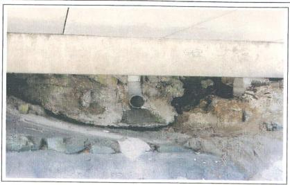
ASSET NUMBER: LOCATION: CULVERT SIZE: CONDITION: 50550 Off Port Road Under Wharf 225mm PVC Pipe PVC pipe exists under the wharf with its outlet surrounded by concrete and rock. No erosion or sedimentation is evident.
