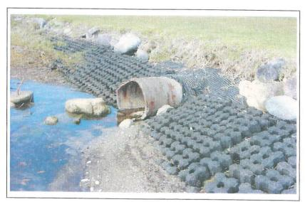
ASSET NUMBER: LOCATION: CULVERT SIZE: CONDITION: 50061 End of Awarua Place 600mm concrete culvert Concrete blocks support the bank around the outlet. No erosion or sedimentation evident. Outlet end is crumbling.
