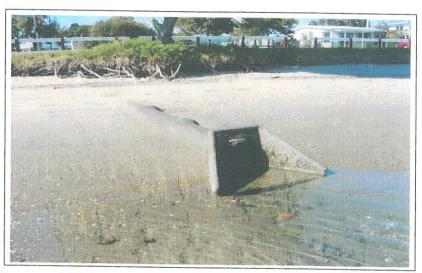
ASSET NUMBER: LOCATION: CULVERT SIZE: CONDITION: 50530 End of Harbour View Road 300mm concrete culvert Outlet extends approximately 5m from the bank. Concrete headwall exists around outlet. No sedimentation or erosion is evident.
