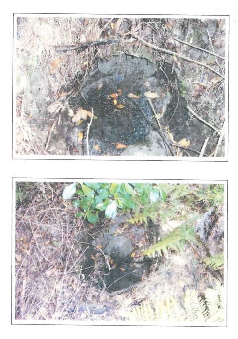
26716 Off Tukere Drive 300mm concrete culvert Concrete culvert outlet in ok condition. SW flows out towards harbour. Banks heavily vegetated. No erosion or sedimentation evident.
