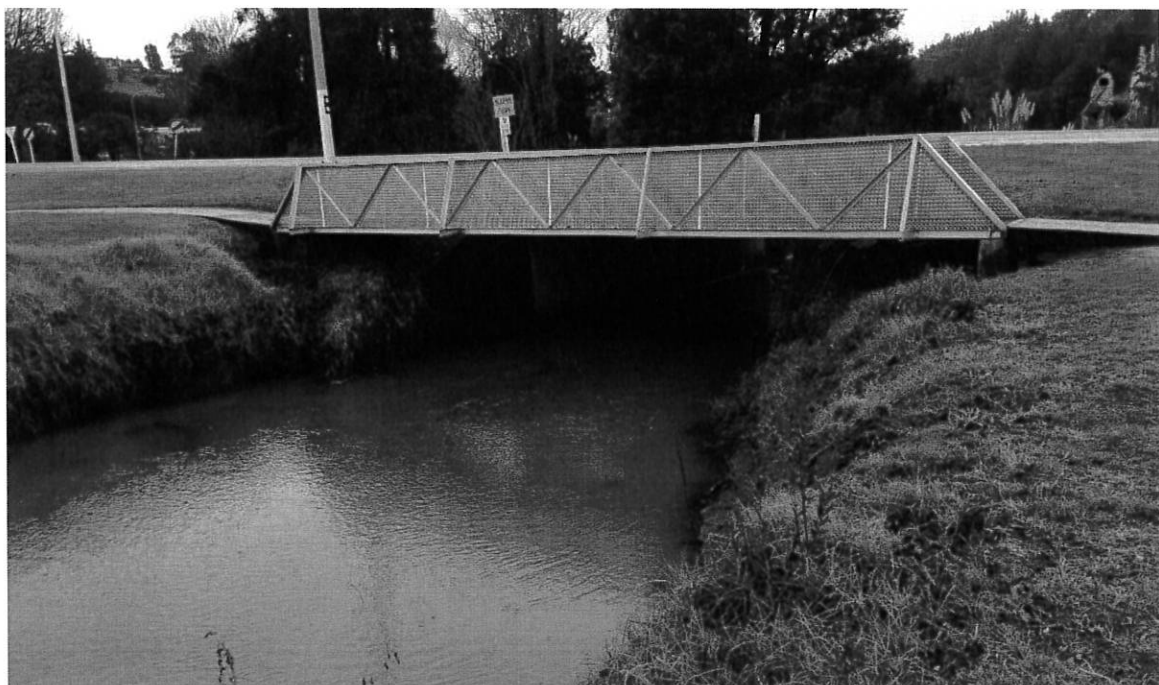
Figure 2-10 SH25 Culvert at Waikiekie Stream
