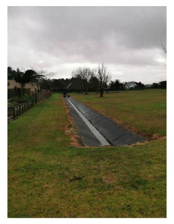
Figure 2-6 Concrete lined open drain at Park Avenue Reserve
