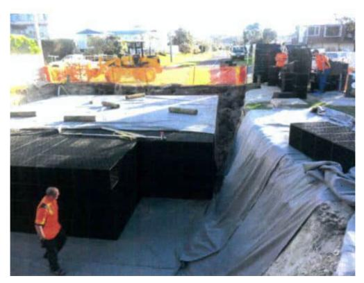
Figure 3-10 Underground storage and soakage near Otahu Road Pump Station
