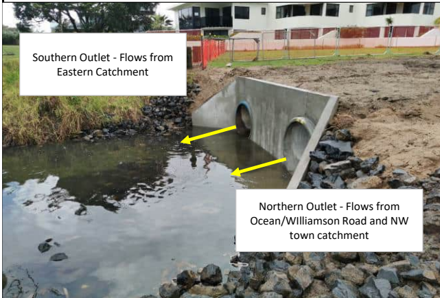
Photo 0 - New 2019 Project - Twin outfall to pond
