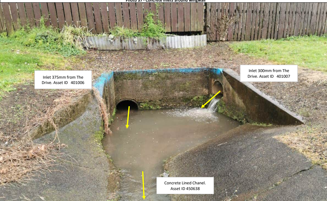
Photo 38 - Concrete Inlets around wingwall - Both appear same diameter
