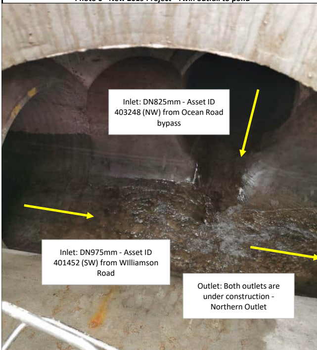
Photo 2 - Inside Manhole above outfall chamber
