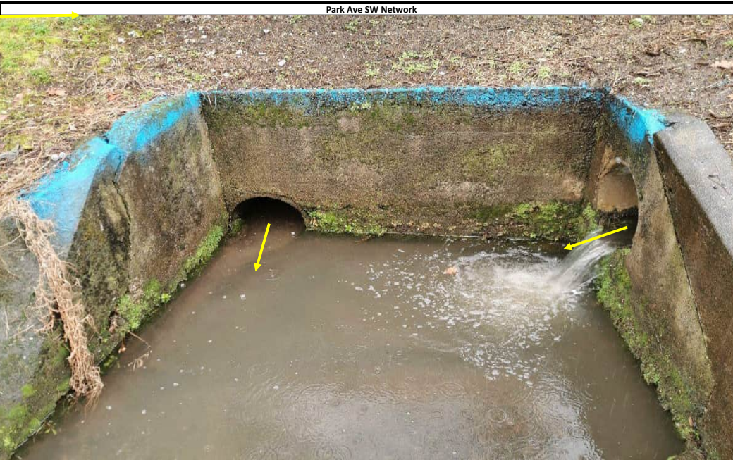
Photo 37 - Concrete Inlets around wingwall
