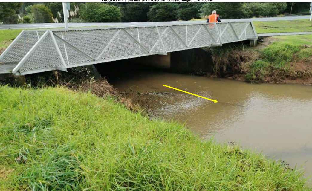
Photo 44 - Size - 2.1m height x 5.5m Width. 3m height total. 0.9 cover
