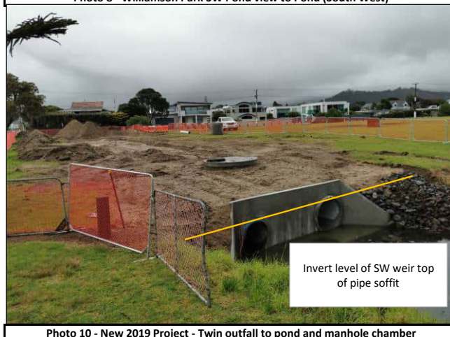
Photo 10 - New 2019 Project - Twin outfall to pond and manhole chamber
