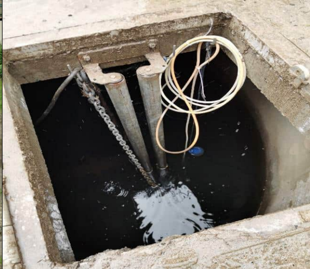
Photo 19 - Otahu SWPS Wetwell - Northern Chamber - 2 Pumps
