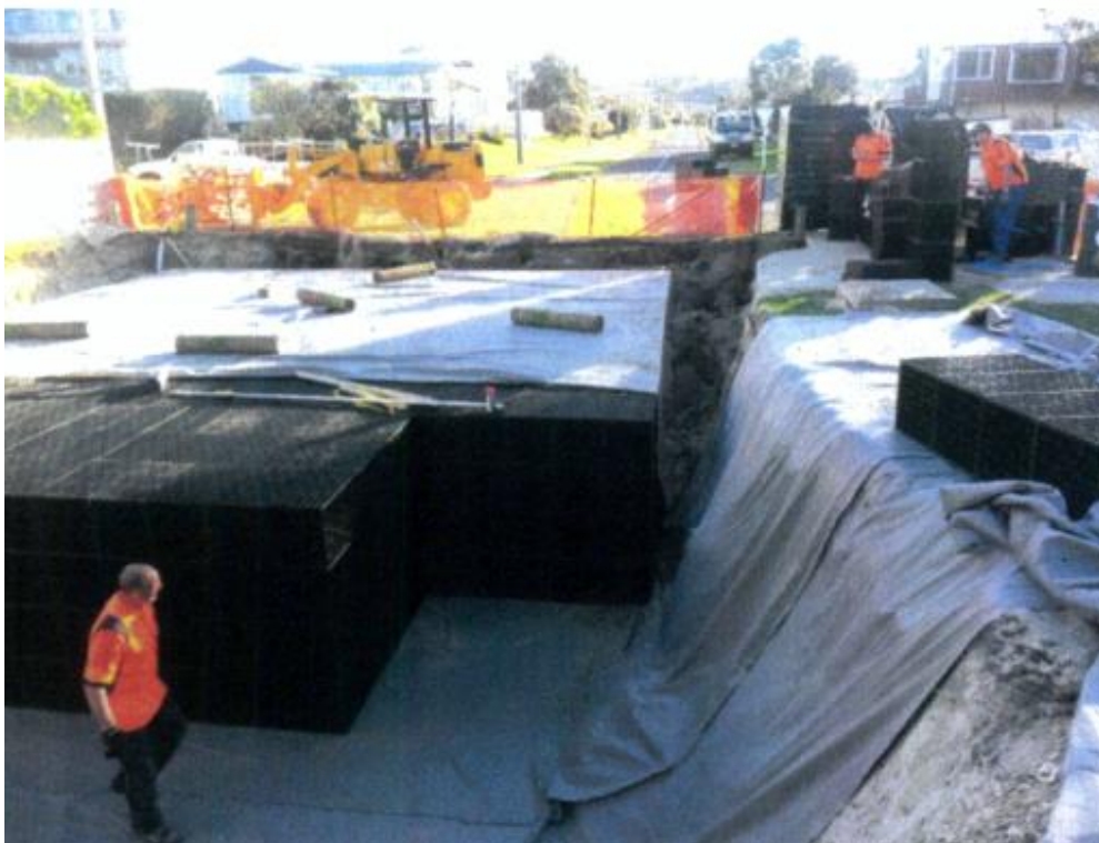
Figure 4-10 Underground storage and soakage near Otahu Road Pump Station
