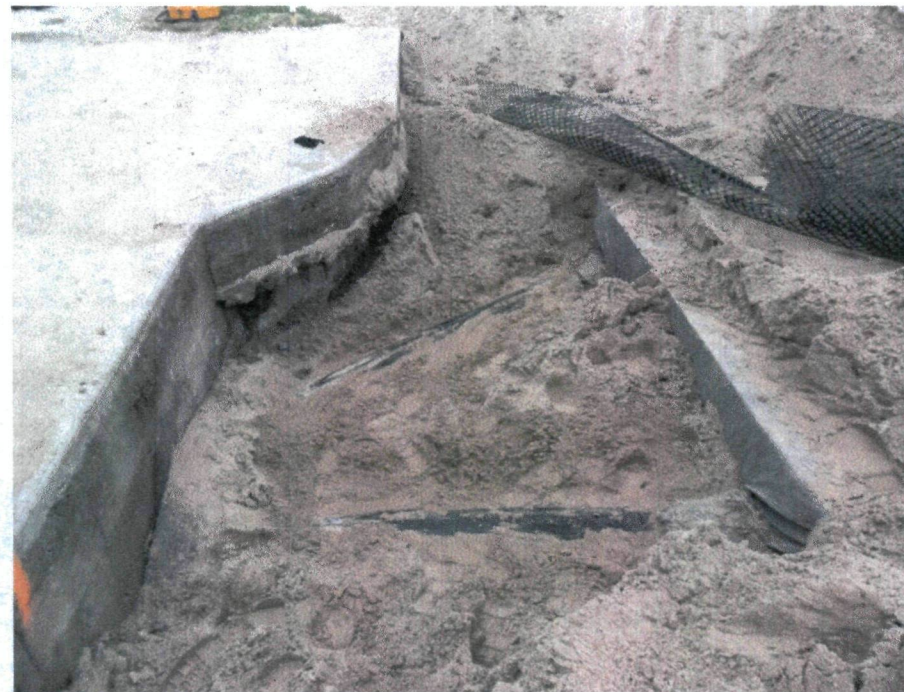
New discharge pipes from the existing pump chamber to the new soakage cells
