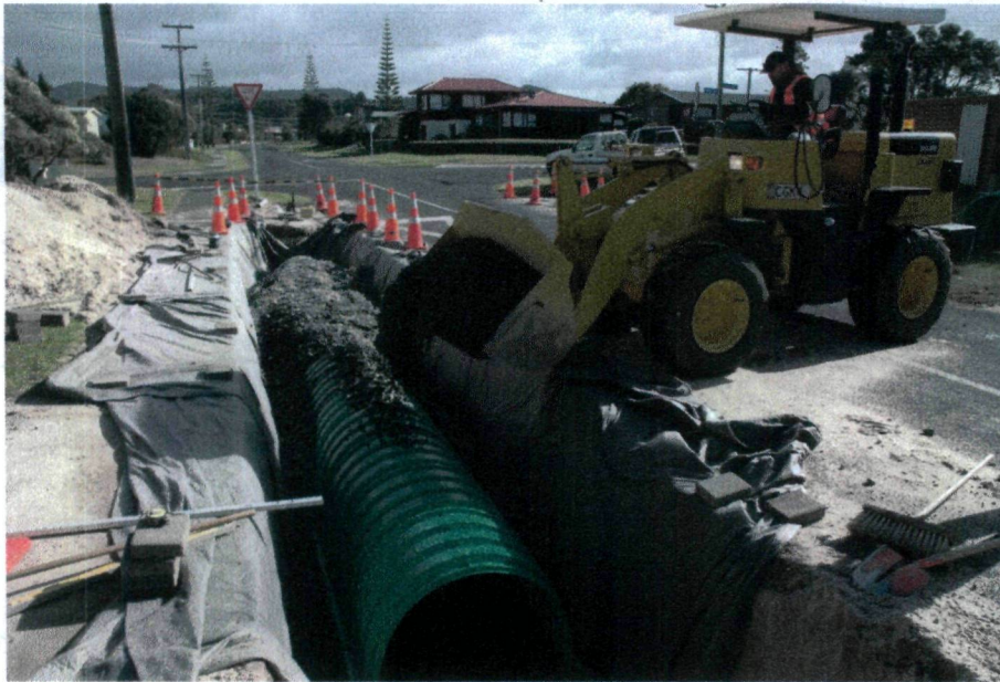
Triton cell - backfilling drainage metal 2/07/12
