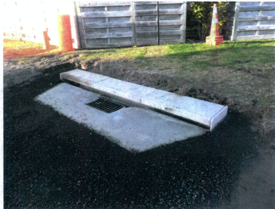
Atlantis cells completed catchpit 28/06/12
