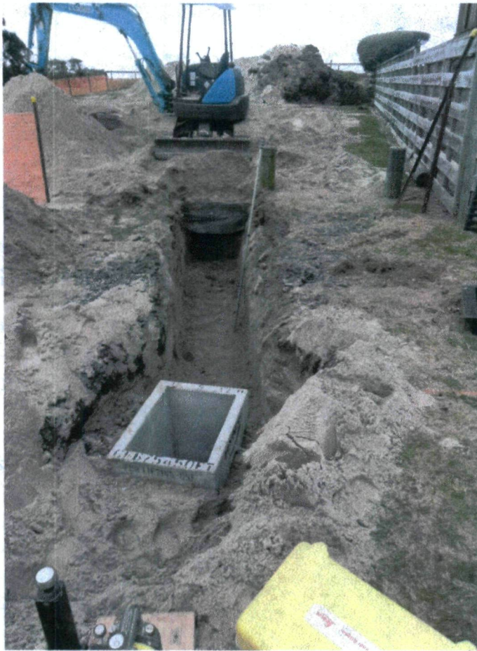
Atlantis soakage new catchpit and lead 18/06/12
