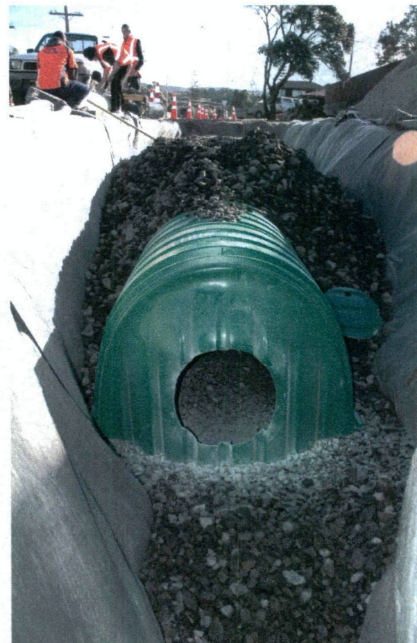
Triton cell end cap at existing sewer bypass 2/07/12
