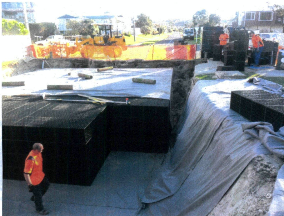
Atlantis soakage cells during construction
