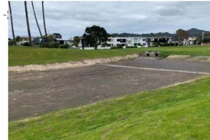
Figure 2: Finished dry detention basin (September 2024)
