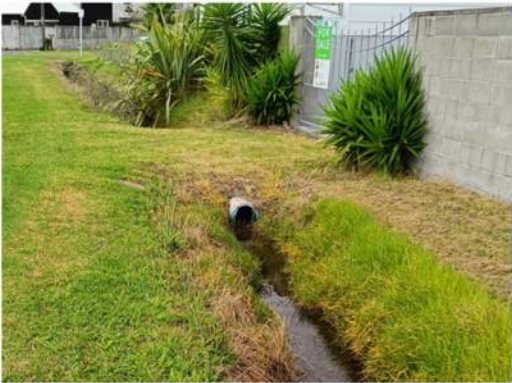
Figure 1: Ponding within the Harbour View swale
